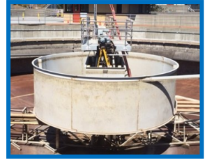
Empty secondary clarifier.
