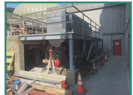
New RDT's being installed.
