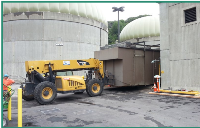
Demolition of the existing DAFs.
