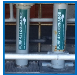
New site sump piping.
