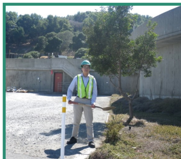
Assistant Engineer, Jacky Wong, at the site of the new Truck Fill Station.
