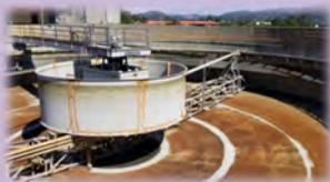
GSE Construction was awarded the project in February, and construction is scheduled to begin this spring. The project includes coating steel surfaces, resurfacing concrete, weir leveling, installation of spray nozzles, and replacing the walkway, the center column, and associated equipment.
