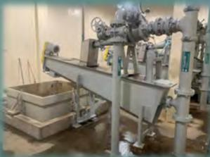
Grit Classifiers are integral to primary solids separation, ensuring inorganic materials such as sand and grit are removed prior to primary wastewater treatment. Due to the nature of their function these units receive a lot of wear, and monthly maintenance is necessary to ensure their upkeep. Because of the continuous exposure to water and erosive grit, despite the regular maintenance, it was time to remove each unit, one at a time, for more involved
