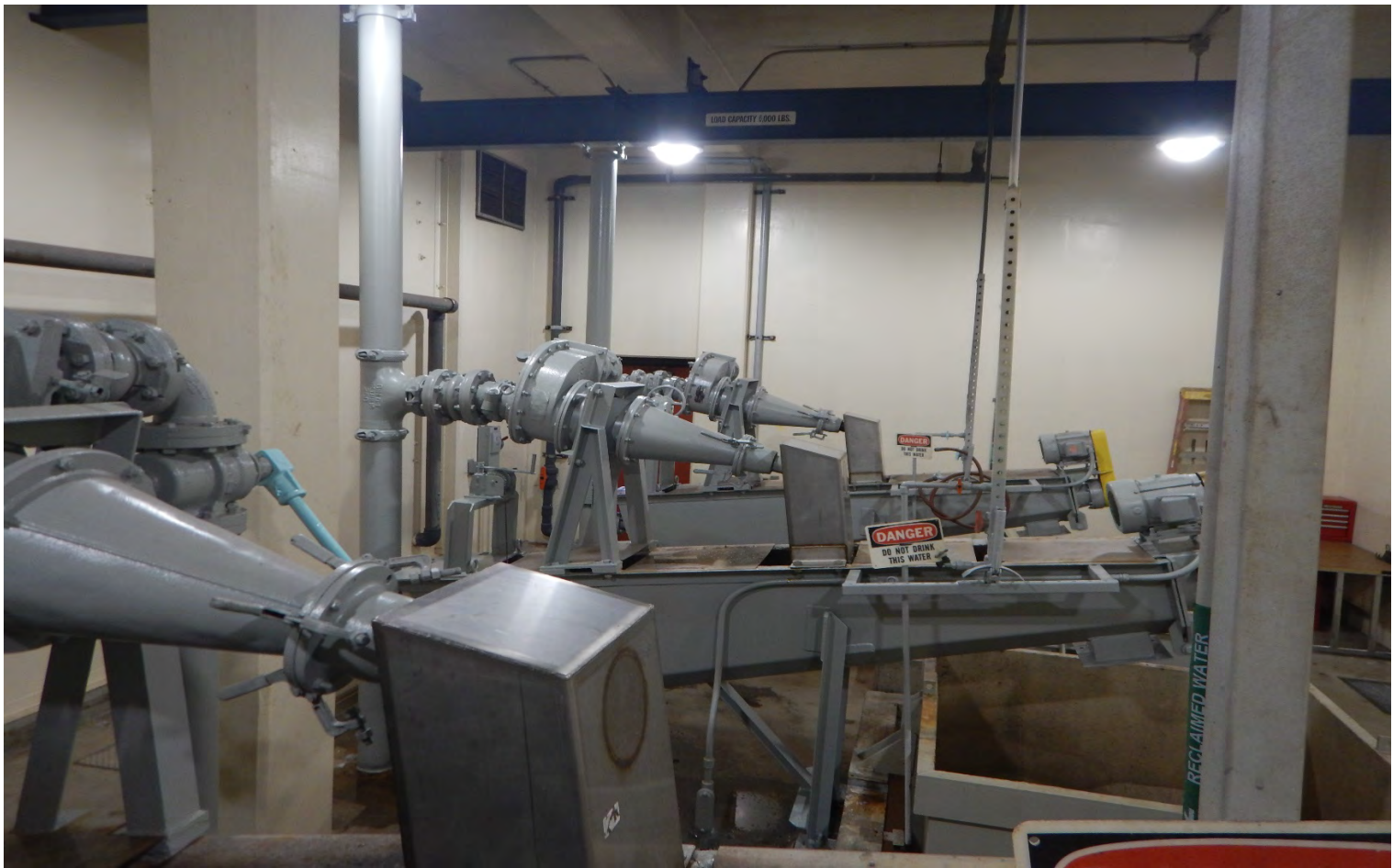
Grit classifiers after refurbishment and coating
