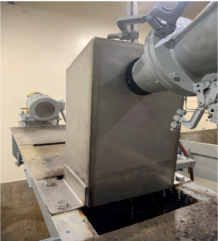
Newly installed stainless-steel grit classifier cover
