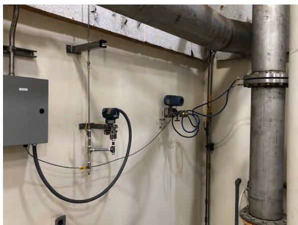
Pressure instrument connected to air piping.
