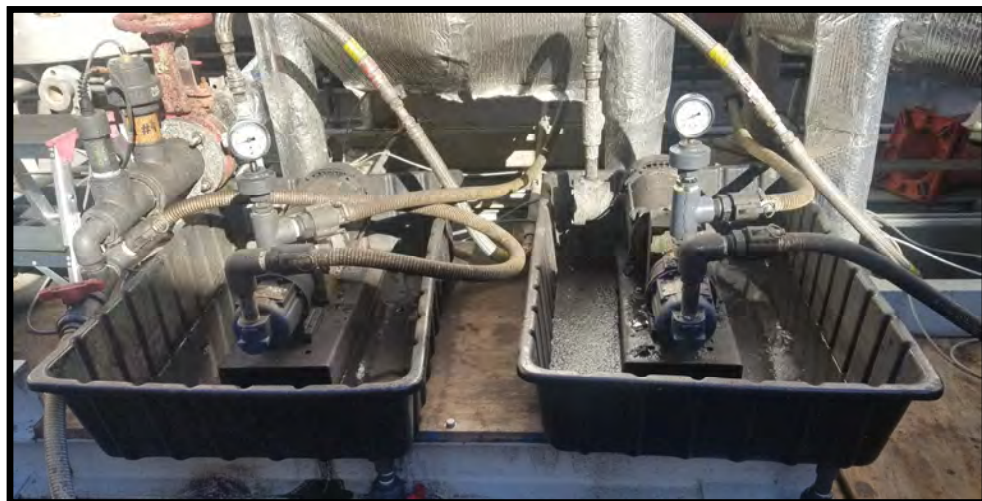
Mix Pump Leaks
