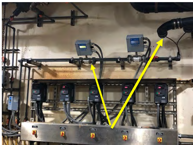
Flow meters and piping to digesters.
