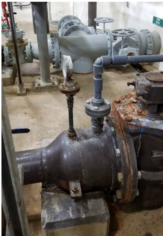
Figure 1: Existing custom-welded fitting on RAS pump suction header
