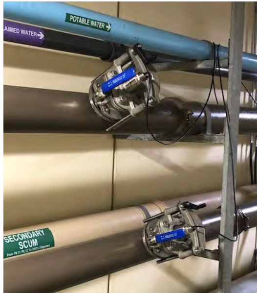
Solids metering probes inserted in piping.
