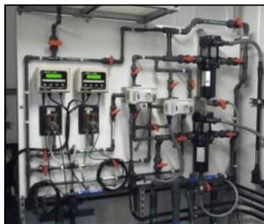
chlorine residual will be discharged to the SF Bay. In the event the second set of analyzers, pictured, senses a small amount of chlorine residual, the SBS Polishing pump will dose a small rate of SBS chemical to ensure a zero chlorinated discharge at a minimal dose. This unit will be tested over the next few weeks in order to fine tune the controls and will be fully functional by the end of April. ♦♦♦
